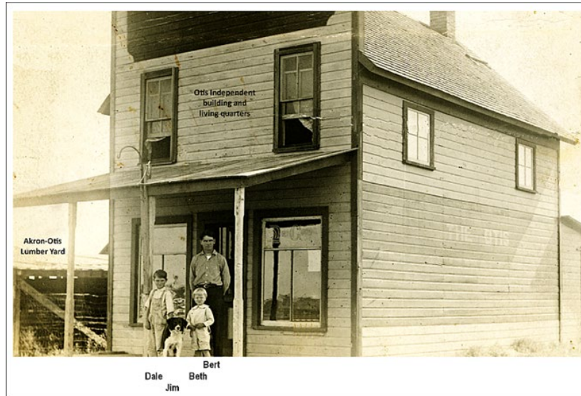
Fig. 7 R.B.. Cooley's first home/business in Otis Colorado
